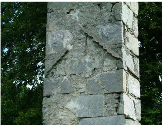
The west face of the chimney showing the 2 lines of flashing
