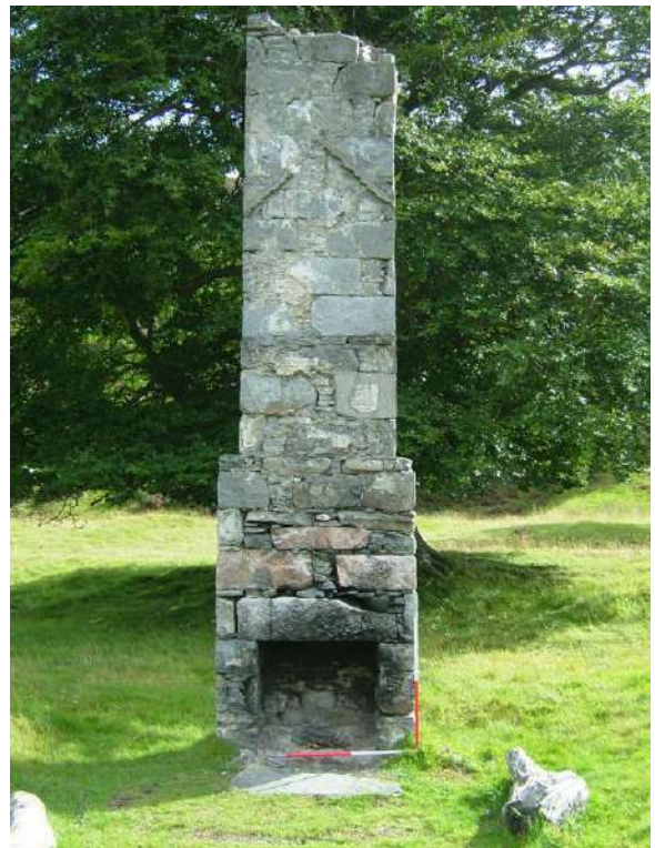
The west face of the chimney
