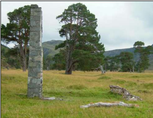
Ruigh Aiteachain - South building with chimney
